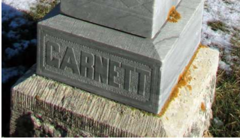
Edge pattern produced by special tool with multiple chisels attached together
