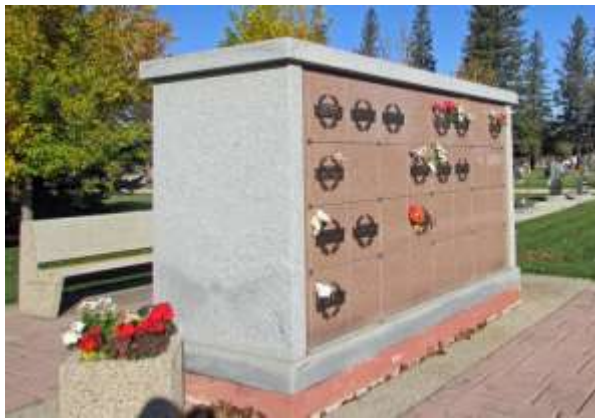
Columbarium (cremation vaults) foundation pads
