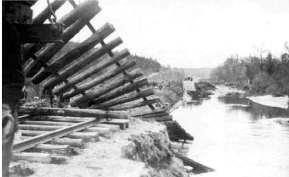
1933 flood destroys railway tracks
