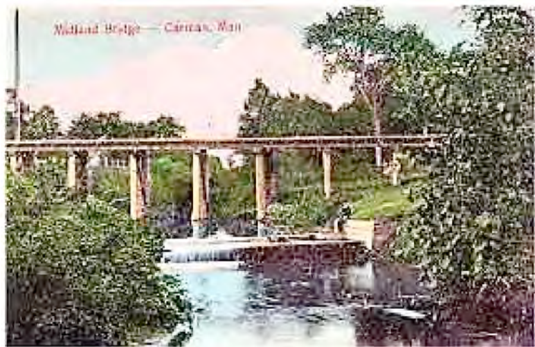
Midland railway trestle
