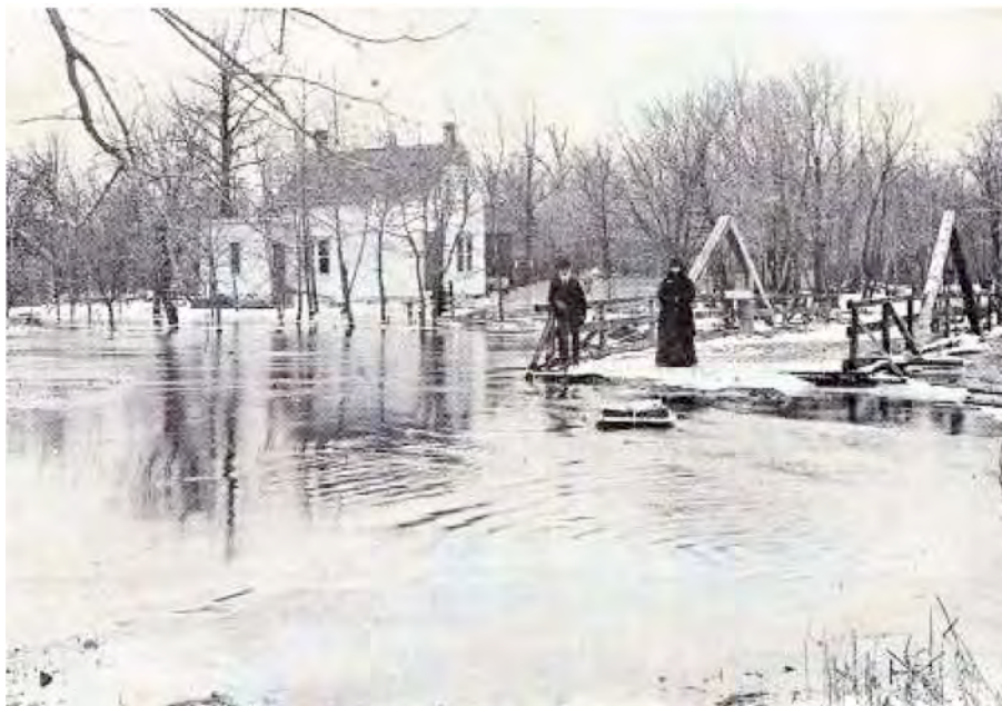
McKnight's Bridge in flood
