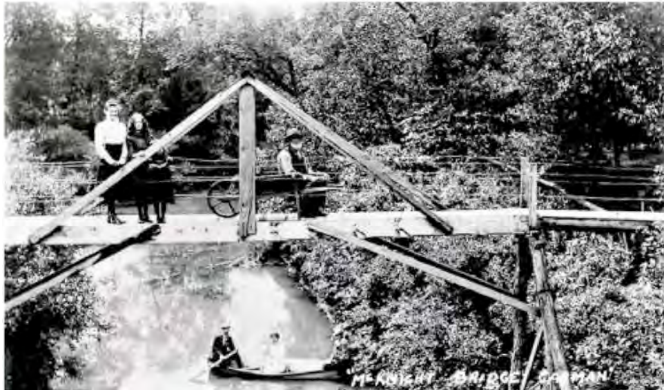
Early McKnight Bridge, near present-day Boyne Lodge.
