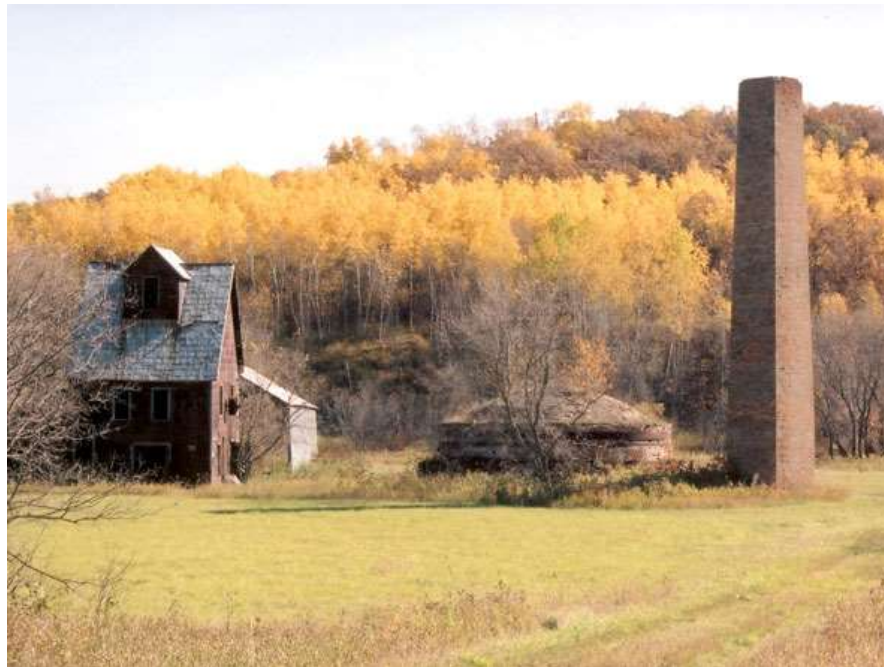
Contemporary view of the Leary Brick Works site, looking to the southwest, and showing the chimney, kiln and on the left the brick plant. The rising terrain in the background, shrouded in autumn foliage, was the site of the shale outcrop used in brick production.
